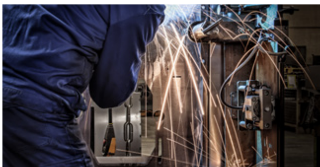
Welding of frame
